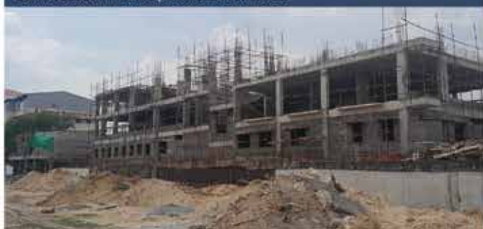
Construction Photo Updated March 2025
